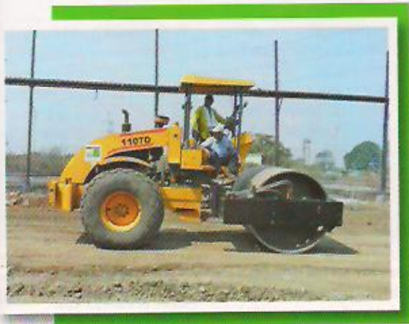
These stabilisers strengthen the base level of soil, thereby ensuring reduction in the bitumen layer.
